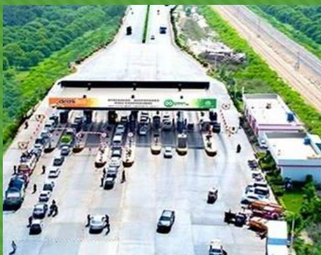
Hyderabad Mirpurkhas Dual Carriageway
